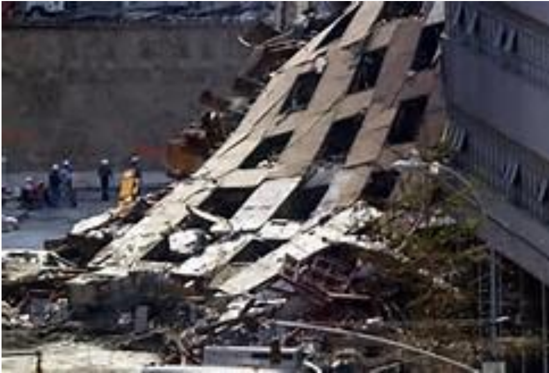
Figure 19 – Concrete Slag of Building 7
