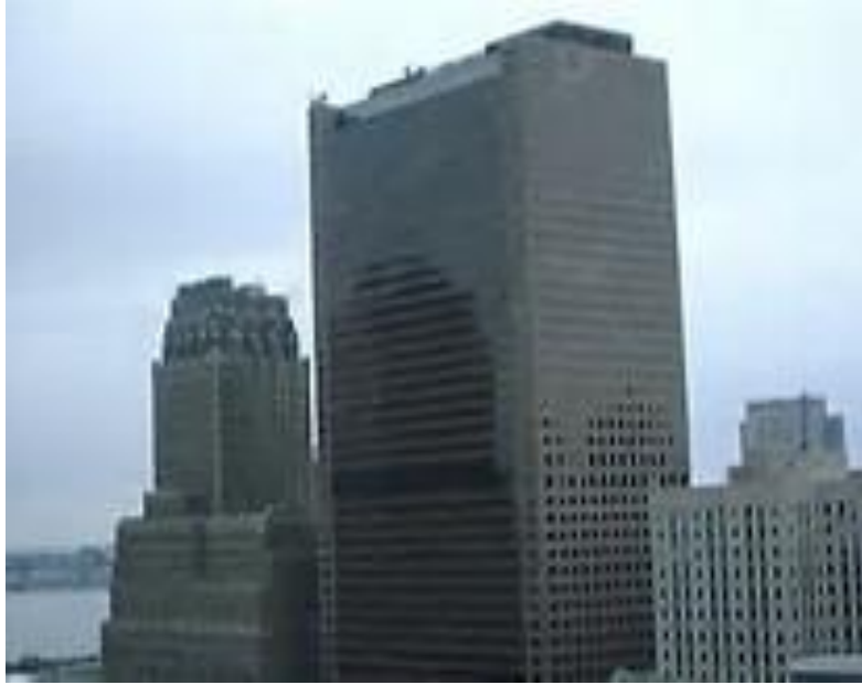
Figure 16 – Building 7 prior to 9/11
